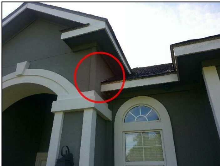
No kickout flashing
