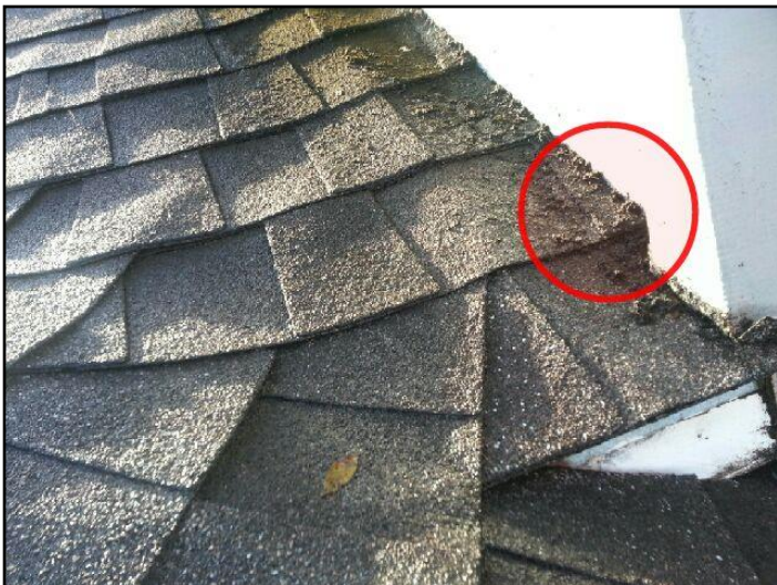
No kickout flashing
